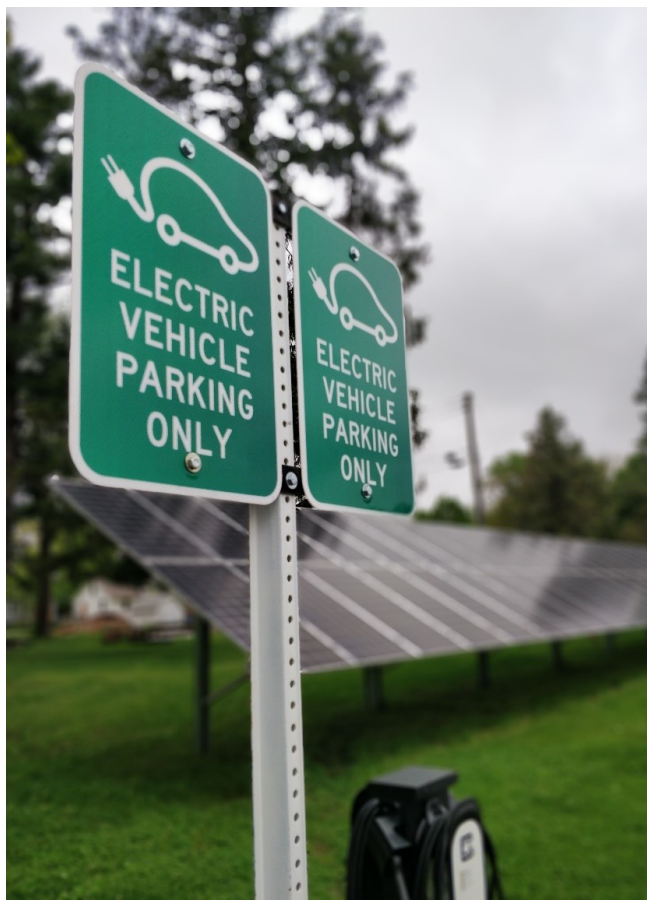
An electric vehicle charging station stands next to solar panels in Iowa. Credit: Jonathan Sundby.
